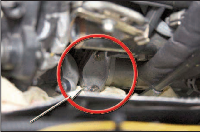
EGR valve blank fitted - indent arrowed!
