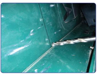
Mark a centre point 6mm in from the corner of the 2 lines and drill a 12mm hole. Repeat this both sides.
